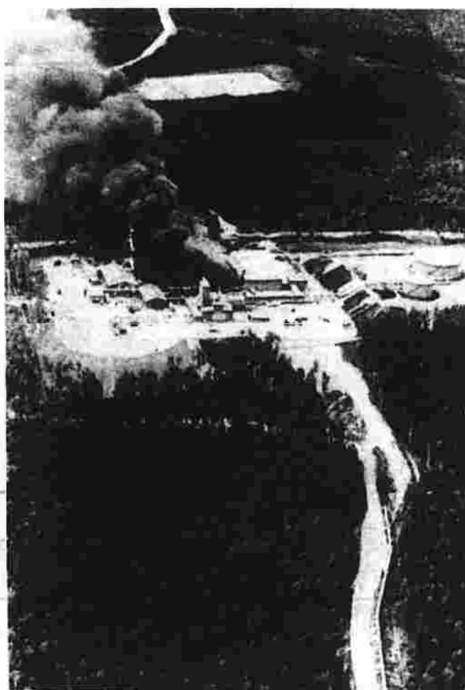
Pump station explosion causes fire This aerial view of Pump Station 8 of the trans-Alaska pipeline shows smoke billowing from a fire which followed an explosion Friday injuring several workers and shutting down the $9 billion system which opened less than three weeks ago. (UPI photo)
